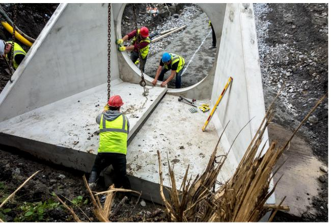
In 2016 P&D Lydon won the contract for the N17 Road upgrade. Tracey Concrete were selected to supply on the drainage products on the Project. XXL Headwalls and DN1800 Spigot & Socket pipes were supplied to the job.
